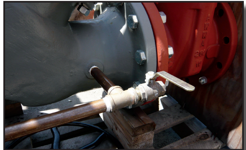
Test Cock No. 4 located on the bypass piping
